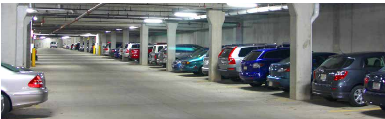
Transition to T8 fluorescent lighting in the Agora parking garage should save the equivalent of 46 tons of CO 2 .
